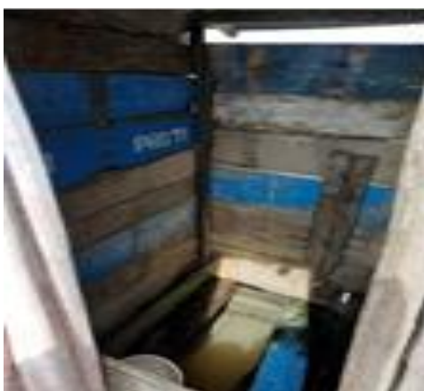
Figure 3. Public sanitation facilities
